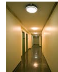
WATERSIDE CORRIDOR PRE-RENOVATION
